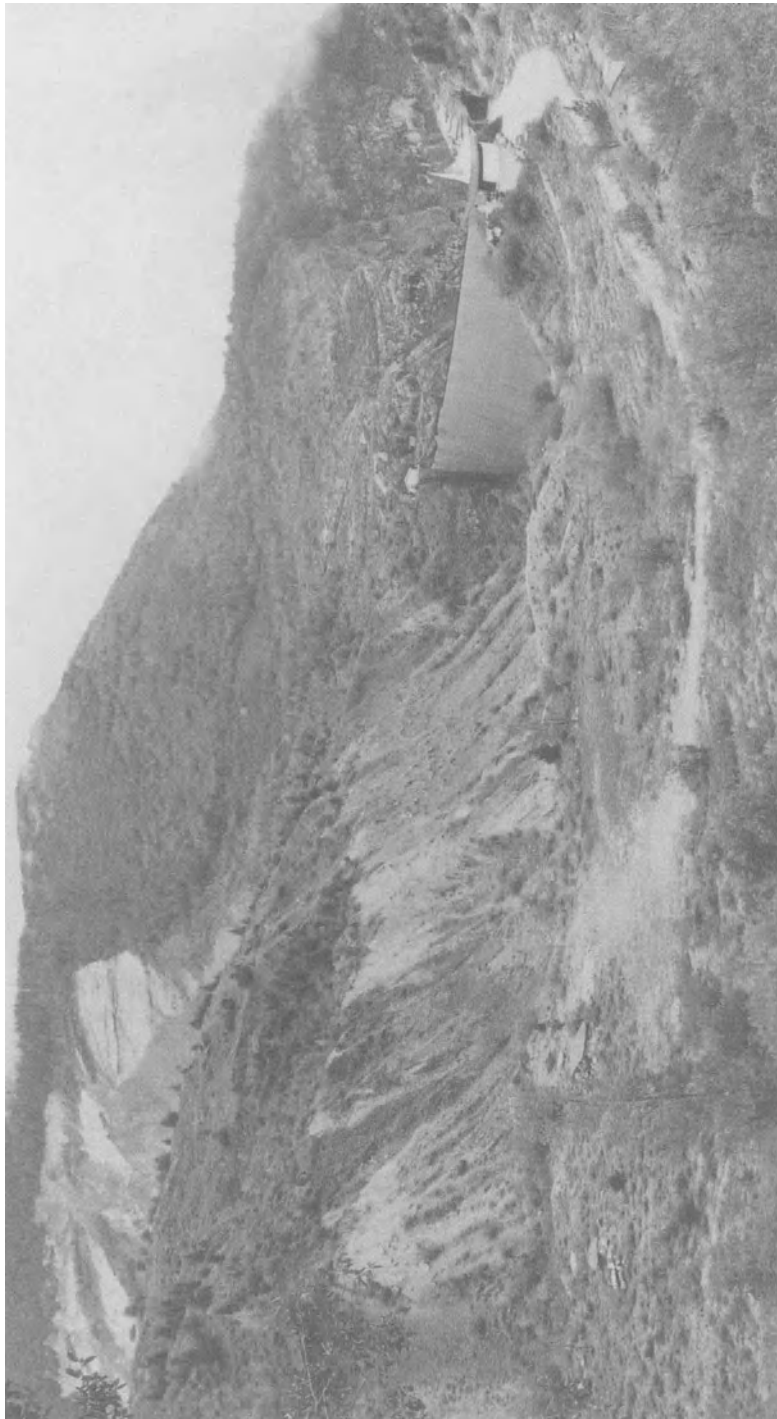
Fig. 2.41. Vaiont rockslide. Practically undamaged dam of the basin. In the background at left the western scar, Photograph, taken in 1984, shows trees of a certain size having subsisted in riding downhill, and younger vegetation witnessing for the humus having remained on top of the mass. Area devastated by water is marked by horizontal periphery reaching from bottom right corner of scar almost to the horizon, then turning downward to disappear behind right end of dam (photo by Erismann)
